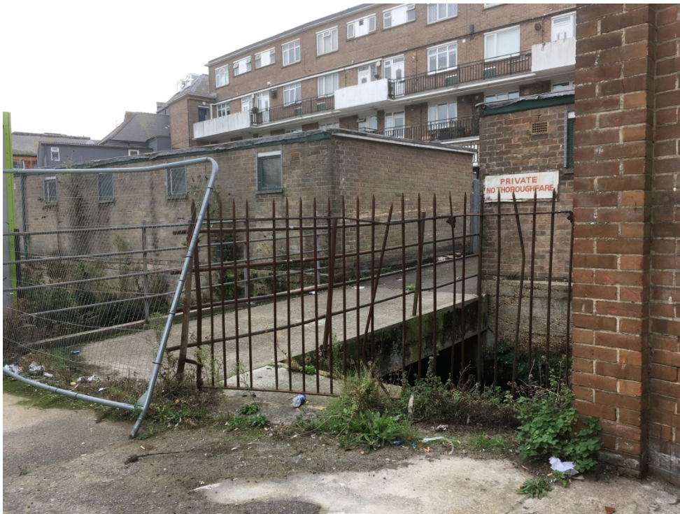
Dolphin House Rear Yard Bridge
